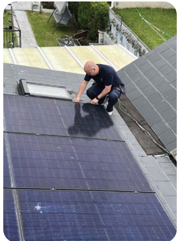
Jonathan on site installing solar panels
